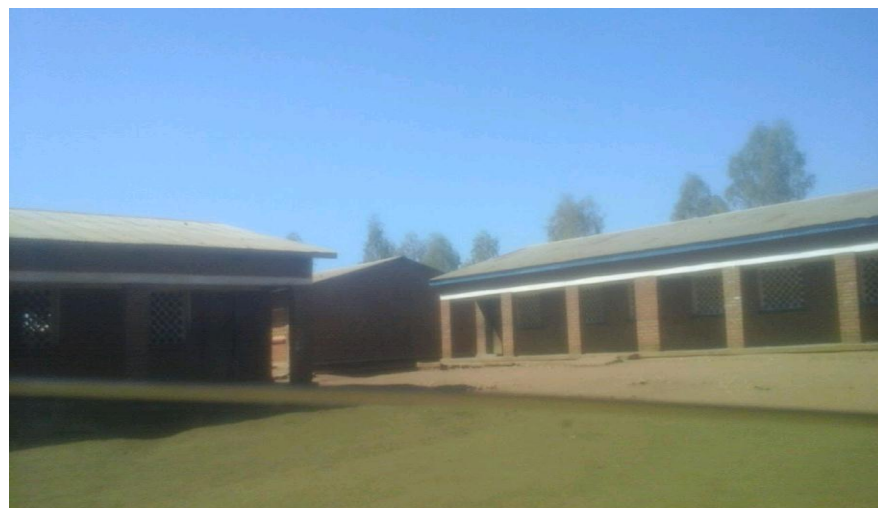
Figure 2: One of the classrooms at School Y
