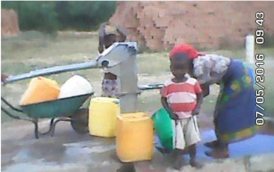
Figure 3: A borehole with a hand pump at School Y
