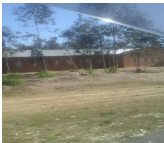
Figure 5: CCAP Church used as a classroom at School X
